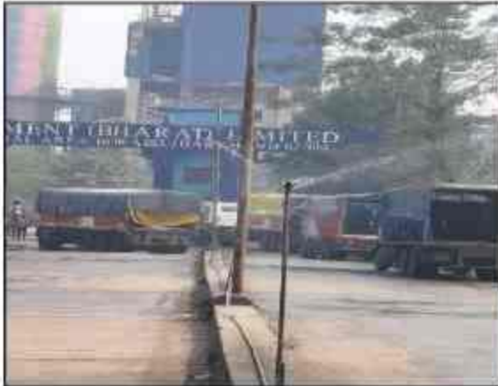
Fixed type water sprinkler installed plant main gate entrance road
