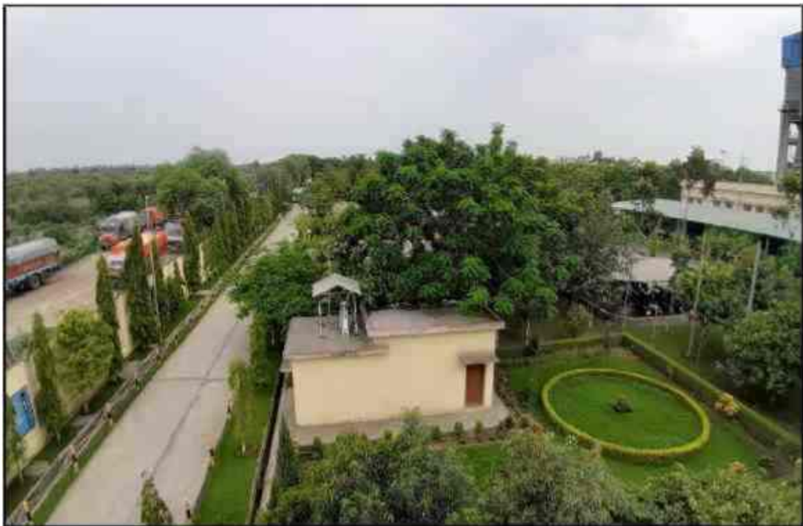
Greenbelt pics at DCBL plant Bokaro
