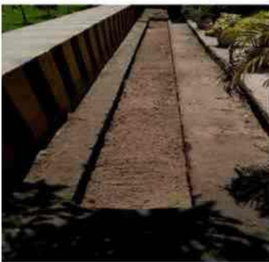
Rainwater harvesting recharge trench near CCR building & near E type quarter
