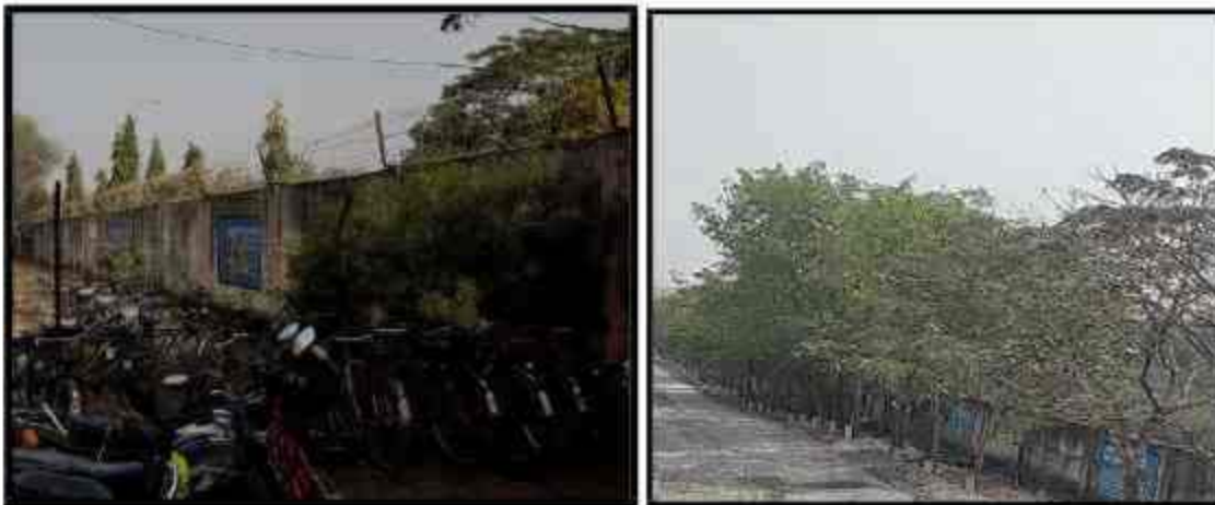
Boundary wall constructed along with tree plantation around the plant
