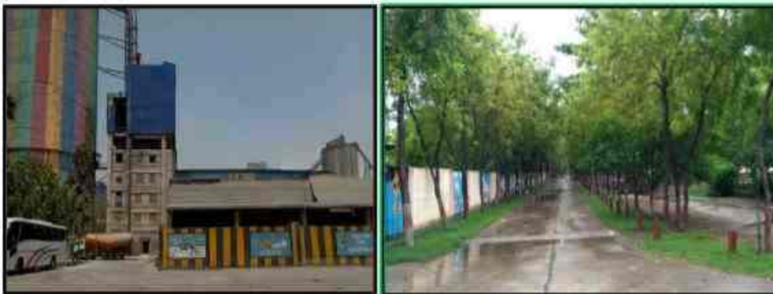
Boundary wall constructed in packing plant area act as wind shelter
