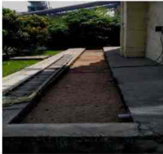
Rainwater harvesting recharge trench near CCR building & near E type quarter
