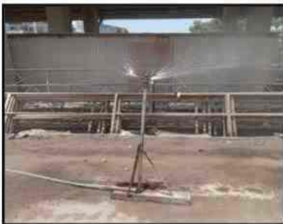
Fixed type water sprinkler installed plant main gate entrance road
