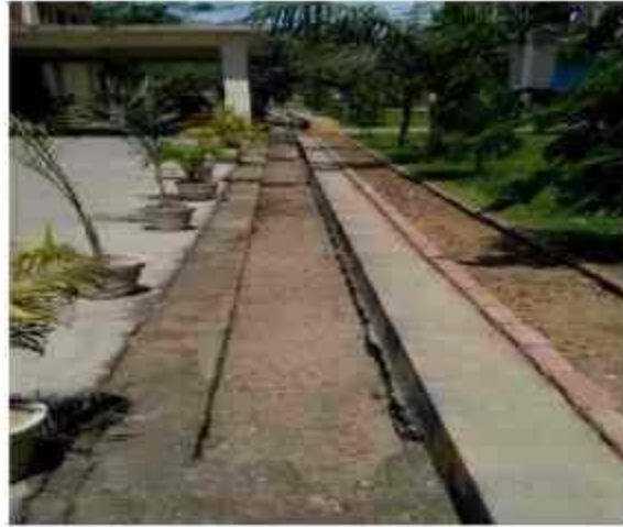
Rain water harvesting recharge pit near FH3 Hostel & Rain water recharge trench In-front of CCR main building
