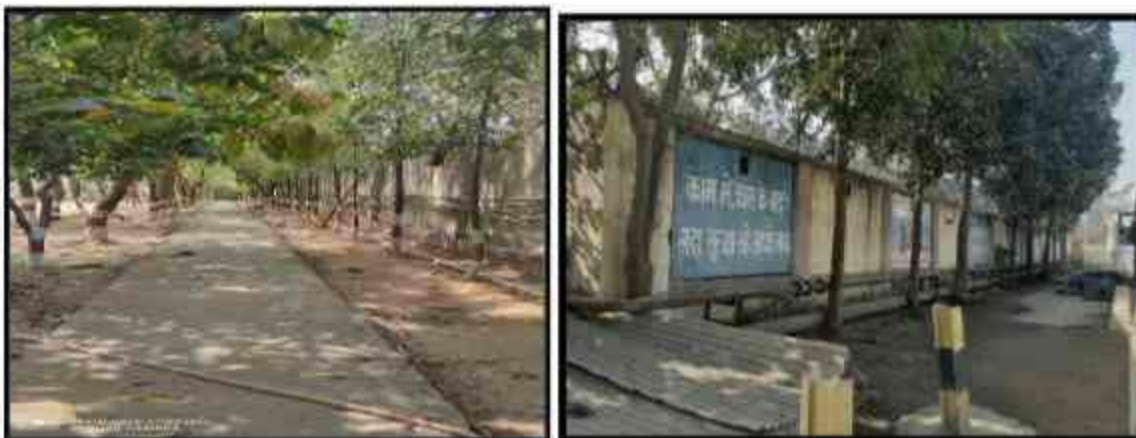
Boundary wall and thick greenbelt developed in between Plant and hostels
