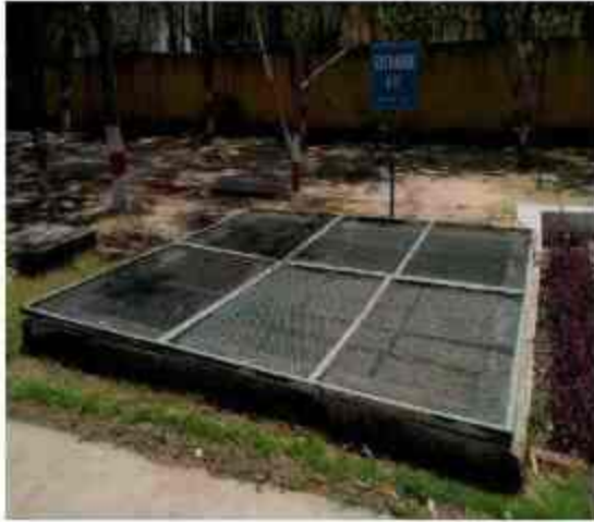
Rain water harvesting recharge pit near FH3 Hostel & Rain water recharge trench In-front of CCR main building
